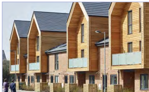
Fig I.19 Effective use of timber brick and slate that complement each other.
