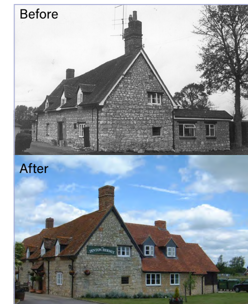
Fig I.2 Successful extension replacing previous inappropriate one.
