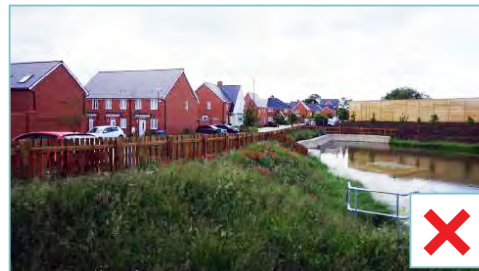
Fig N.13 Attenuation pond is poorly integrated resulting in limited visual amenity value.
