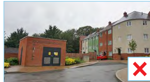
Fig B.22 Sub- stations that are free standing and prominent at the ends of the street adversely impact the residential environment.
