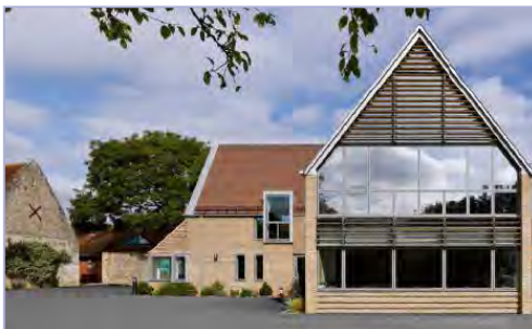
Fig I.18 Modern materials reflect adjacent existing building.
