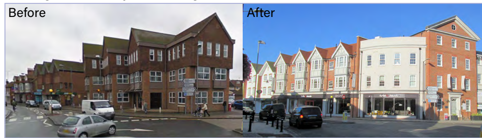
Fig I.3 Successful replacement of inappropriate 1970s building in Marlow by referencing local character.
