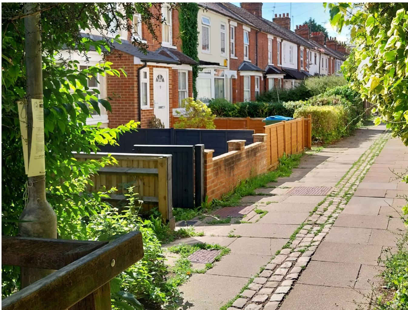
Replaced boundary treatments along Highbridge Walk
