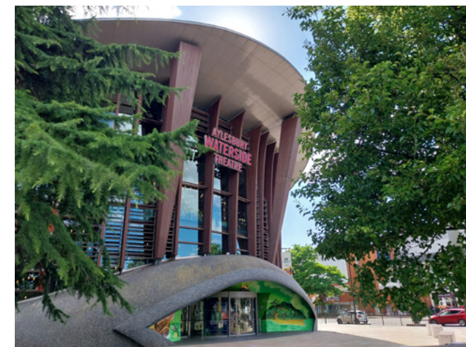
The Waterside Theatre
