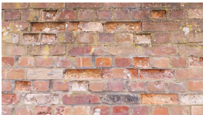
Brick that has worn away due to moisture being trapped within the wall because of cement mortar pointing
