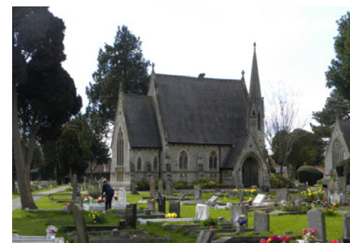
Chapel in Tring Road Cemetery (1856-1857)
