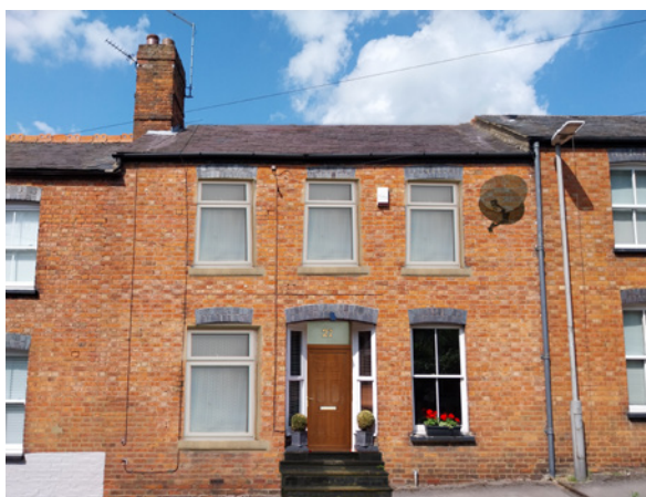
The alteration of original design features in renovation projects, such as the opening of the central blind window and removal of decorative ridge tiles when re-roofing, remove the building's finer architectural features.
