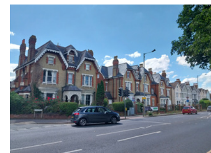
Wendover Road villas are immediately experienced from the road, with their high-quality frontages clearly visible
