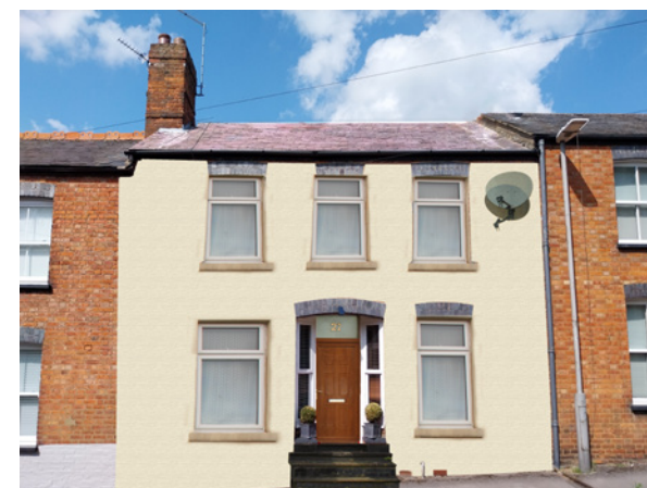
Painting or rendering of masonry walls and replacement of historic door and fanlight in a modern style cover any sense of the building's historic appearance and its relationship with surrounding buildings. The loss of a redundant chimney stack further throws the building's symmetry out of balance.
