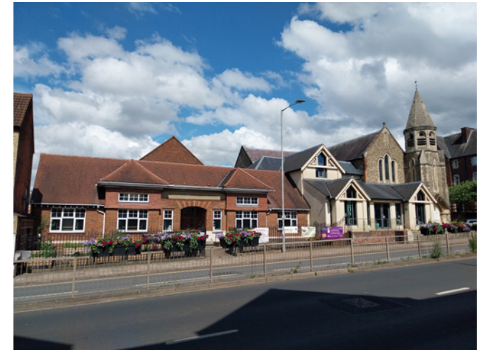
Holy Trinity Church and Parish Hall in Walton
