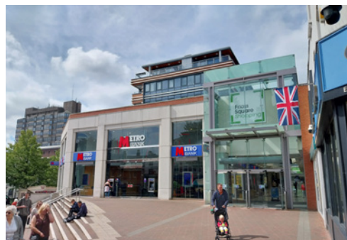
The monolithic Friars Square shopping centre directly adjacent to the Conservation Area boundary
