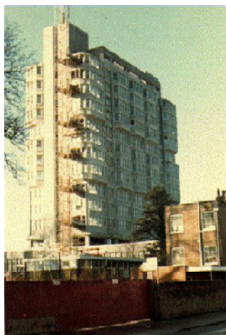
The New County Offices under construction, 1966 (Buckinghamshire Archives)
