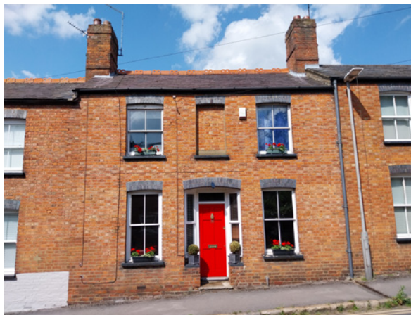
A late-Victorian red brick terrace that retains its original symmetrical composition and features, including sashes, six panel door and blind window.
