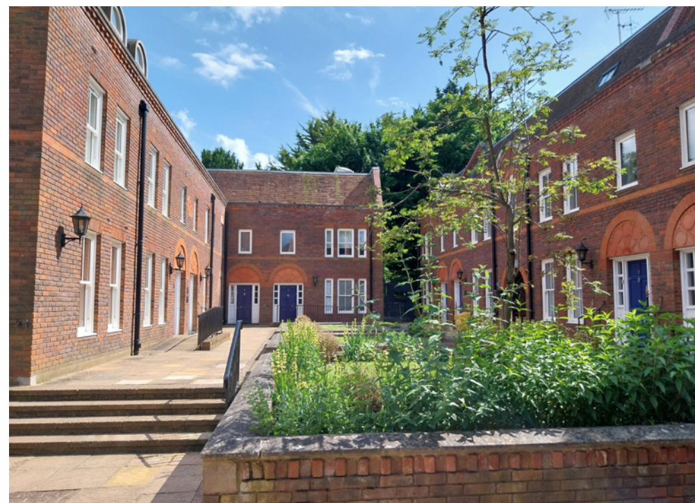
Courtyard-style residential development at Prebendal Court, which uses modern design that picks on traditional forms and features such as sash windows, with bespoke details like terracotta moldings
