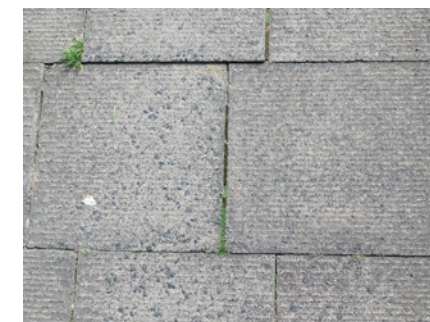
Concrete slabs common on pavements
