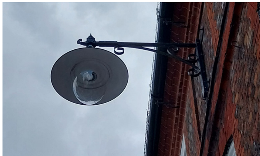
Attached historic-style street lighting on Castle Hill and Temple Street
