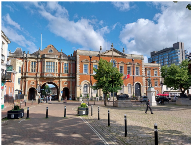
View of civic buildings at the southern end of Market Square
