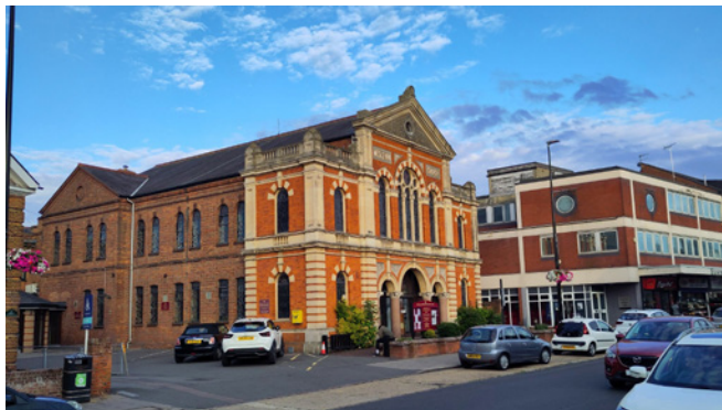
View 04: View of the prominent Methodist Church, dominating Buckingham Street on approach from the north
