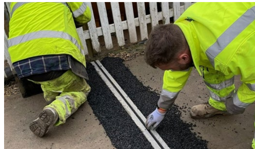
Figure 25: Buckinghamshire Highways installing in-pavement channel in Wendover
