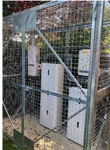
Figure 17: Aylesbury Family Figure 17: Solar PV & battery storage at Hazlemere Library Time Centre
