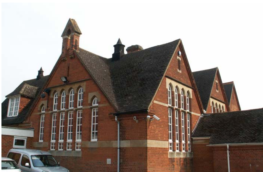
The school showing the empty bell cote, the elegant lancet windows and multiple steeply-pitched gables.
