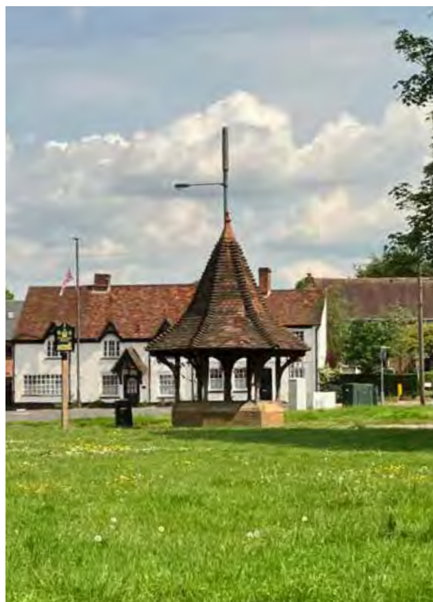
Figure 06: The Pump Shelter, Farnham Park
