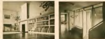
HOUSE AT FARNHAM COMMON
