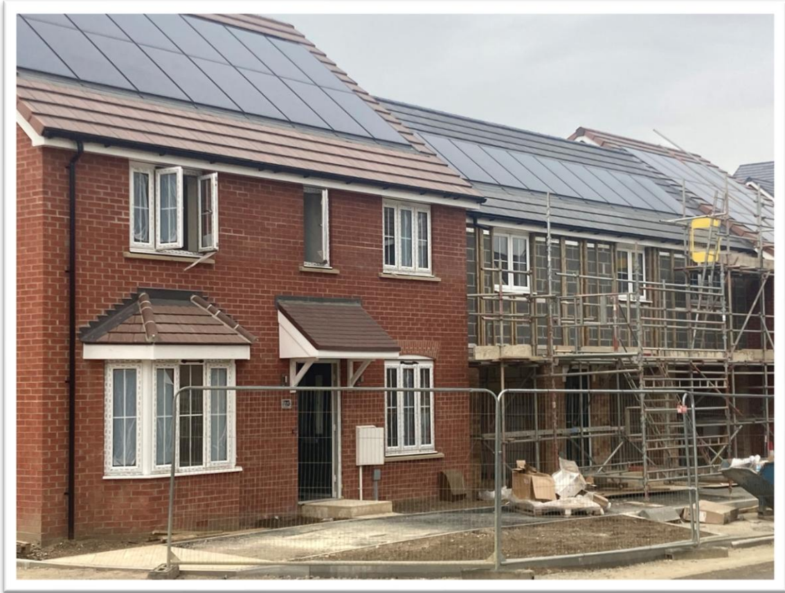
New build with roof solar panels
