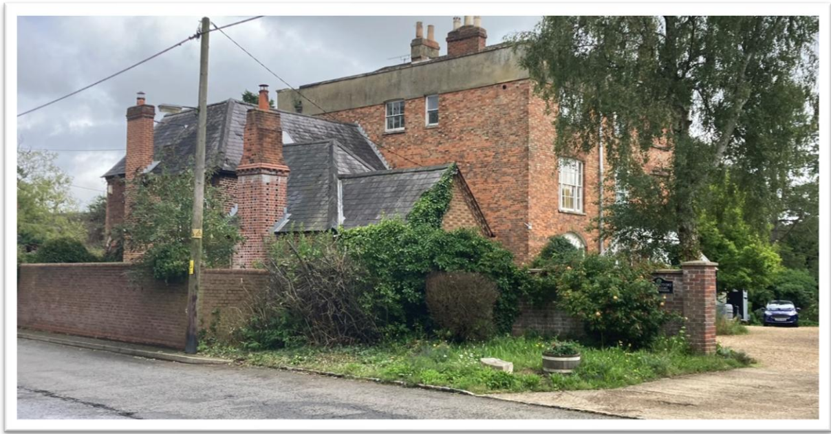
The Grade II listed Flat, the Old Parsonage and the Old Rectory, Drayton Road
