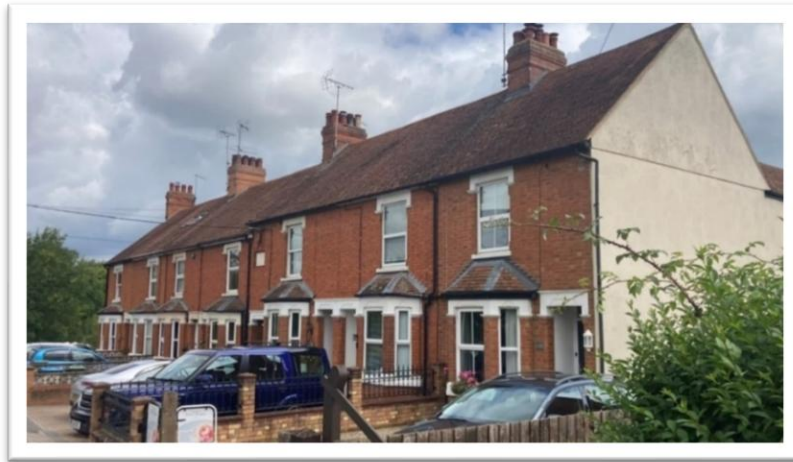
Brickworks cottages, 108-120 Bletchley Road
