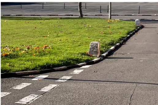
Opportunity to reuse existing internal streets where appropriate and retain black and white kerbs where possible.
