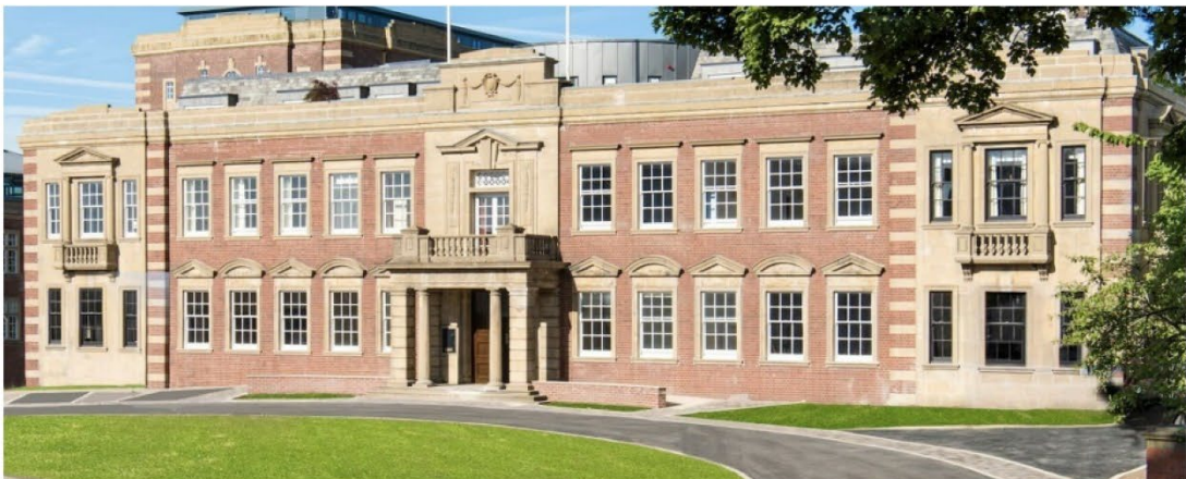
Former chocolate factory renovated into care home. Chocolate Works Care Village, York
