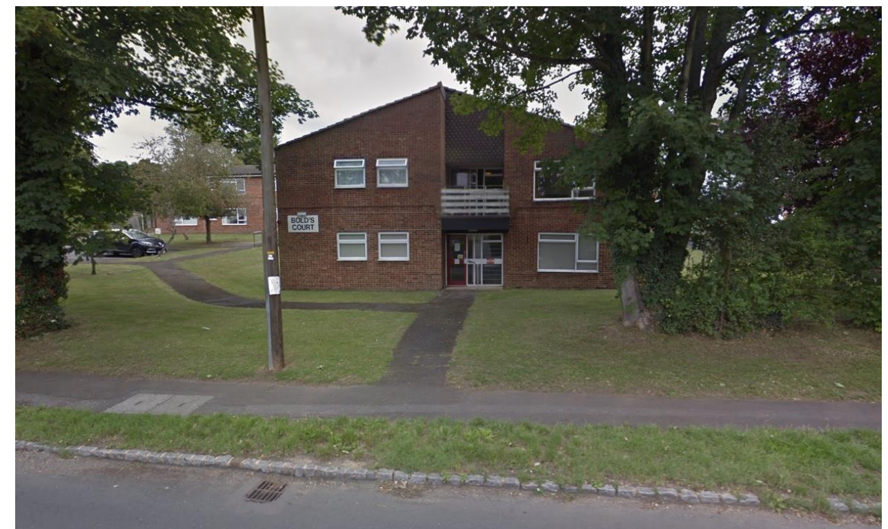
Site frontage to Rogers Lane
