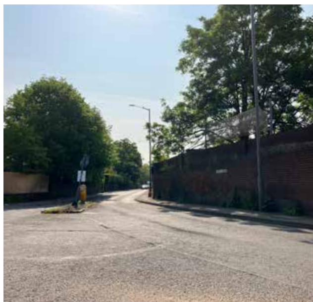
Figure 25: B416 - Stoke Green Junction.
