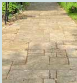
Permeable block paving
