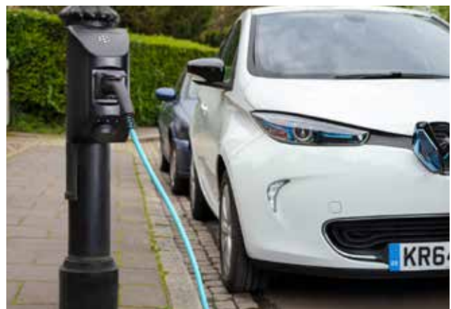
Figure 59: Example of on-street electric vehicle charging points.
