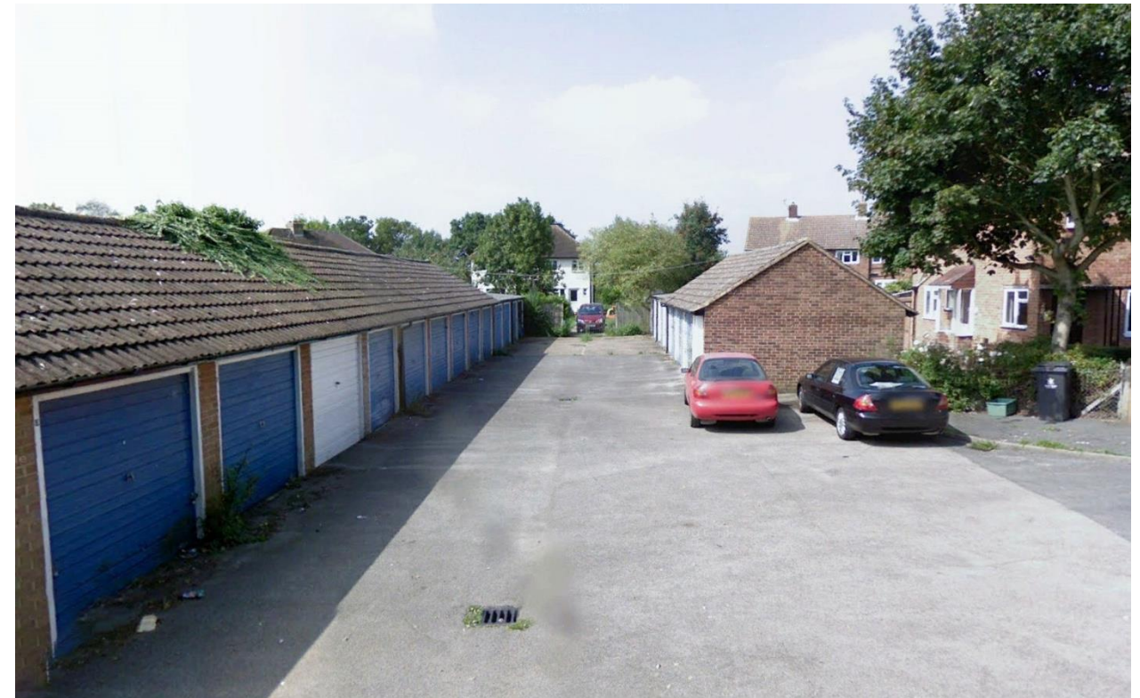
Existing row of garages within the site
