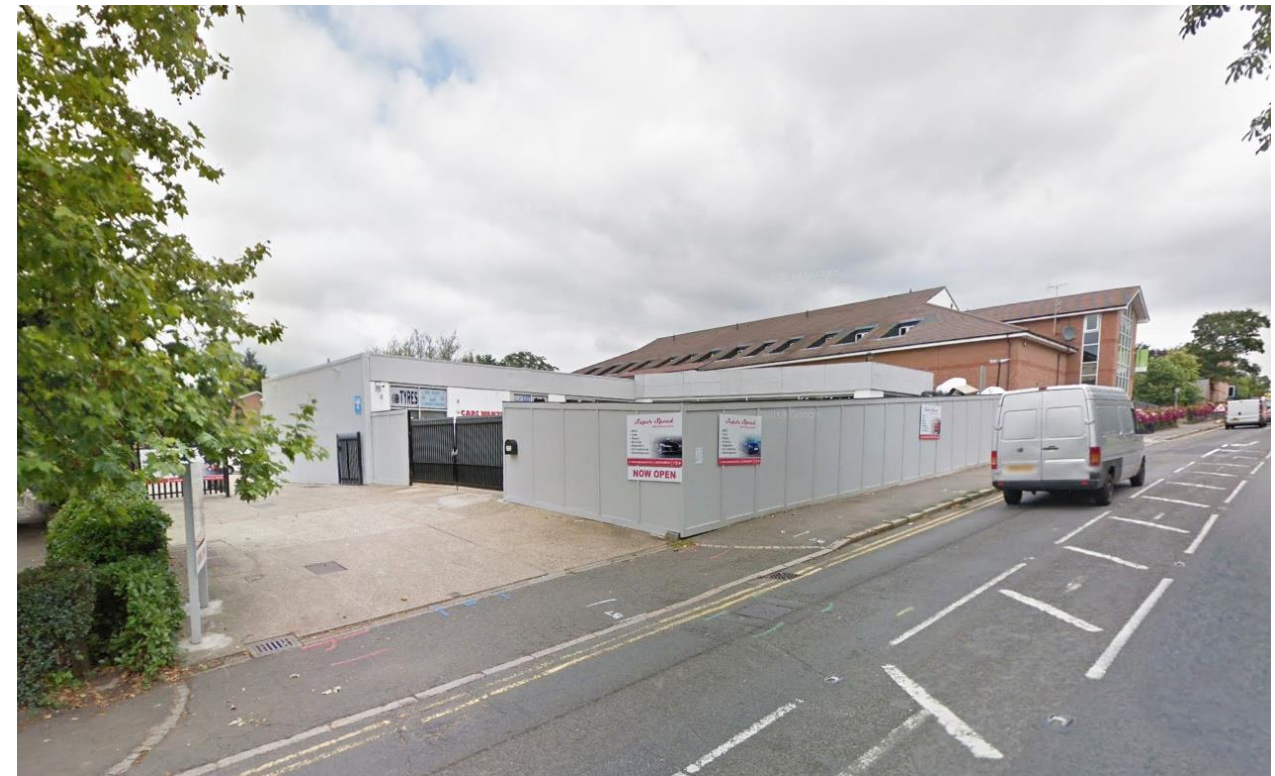
Site frontage to Bells Hill
