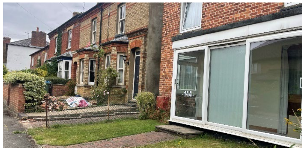
Figure 47 An inappropriate front porch extension
