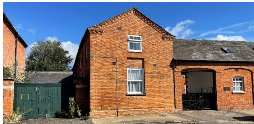
Figure 48 uPVC windows and rooflights in Horn Street
