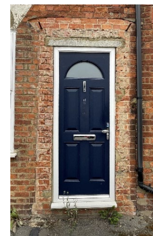
Figure 46 Removal of architectural detailing and inappropriate materials
